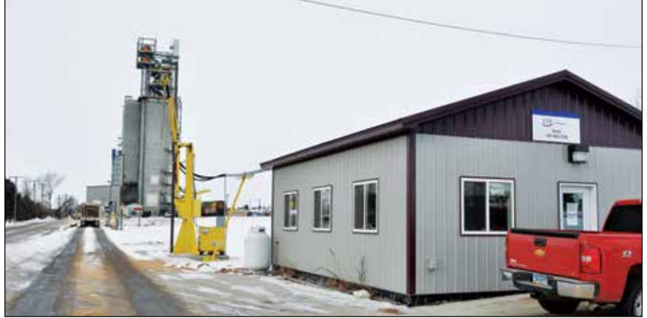
Scalehouse and new Gamet Apollo probe station outside the Garrison elevator. Truck is parked on a new Rice Lake inbound scale in distance at left.
