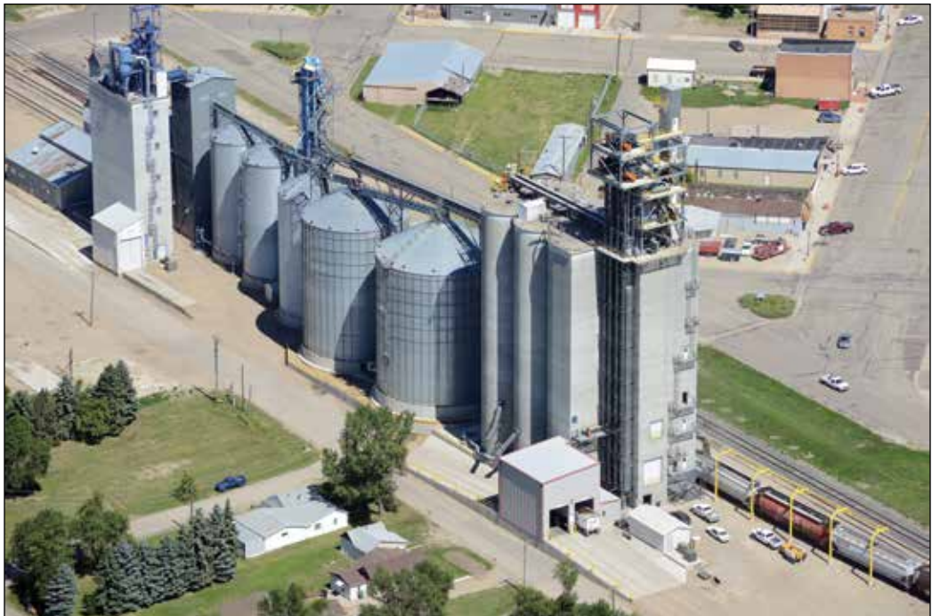
CHS Garrison flagship facility in Garrison, ND, with new slipform concrete annex at right. Aerial photo courtesy of Vigen Construction, Inc.
