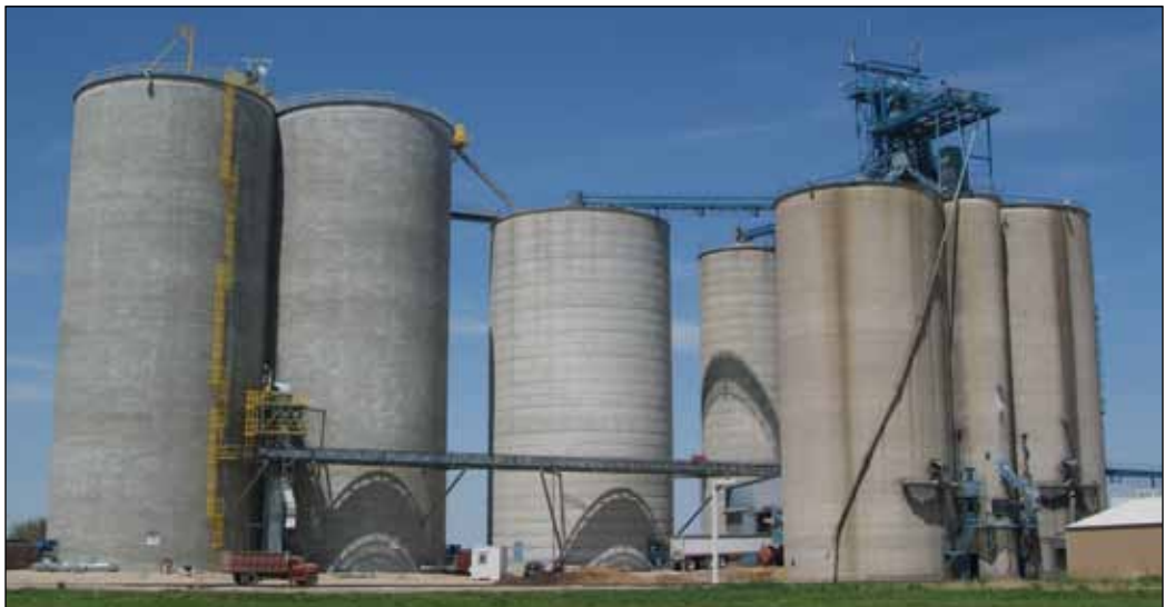
The two new tanks at Grand Island, NE are at the left end of the facility. Also visible are a 30,000-bph Schlagel jump leg for unloading onto an overhead Hi Roller enclosed belt conveyor.
