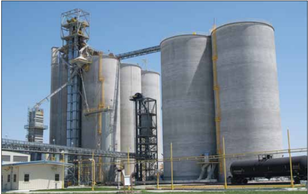
The grain elevator portion of Aurora Cooperative Elevator Co.'s Aurora West complex near Aurora, NE includes two new 294,000-bushel slipform concrete tanks at right. Photos by Ed Zdrojewski.
