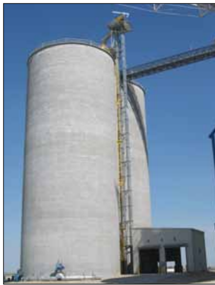
Two new tanks, twin receiving pits, and receiving leg at Aurora Coop’s country elevator in Sedan, NE.
