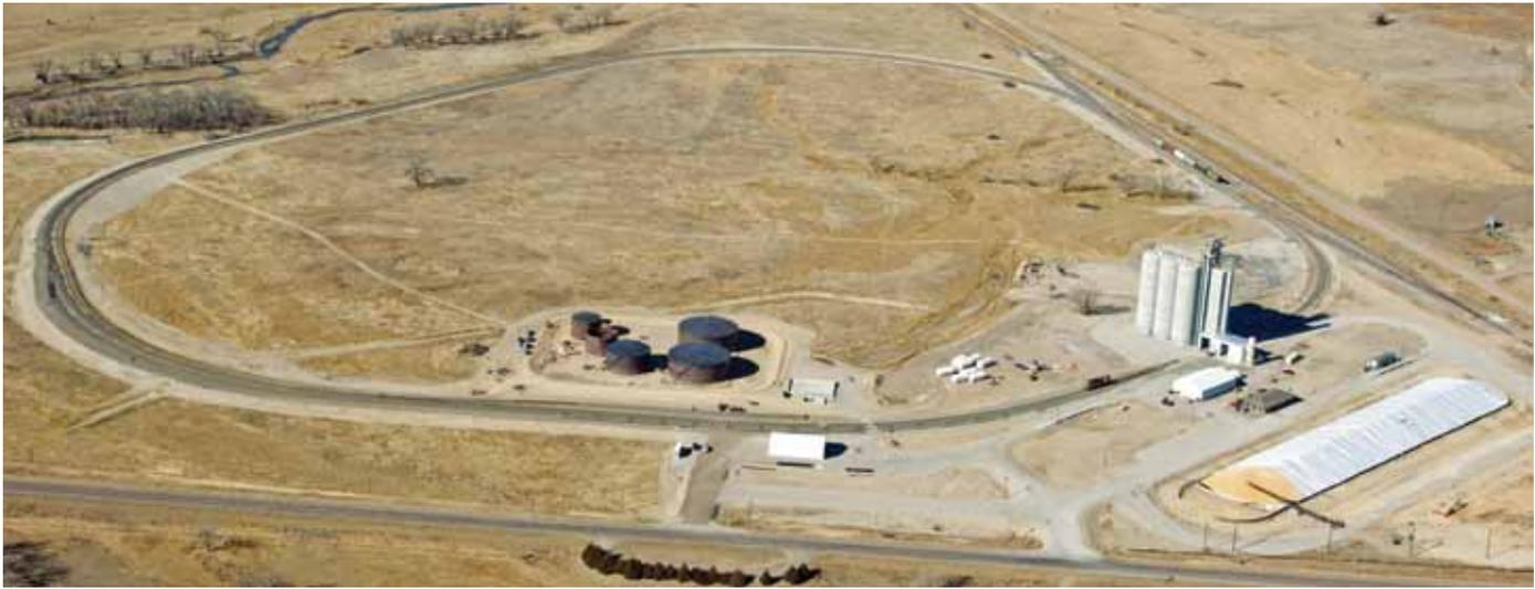
*The new terminal has more than 11,000 feet of track including a loop track off the Burlington Northern Santa Fe for nonstop rail loading. Photo by Heaven's View Photography.*
