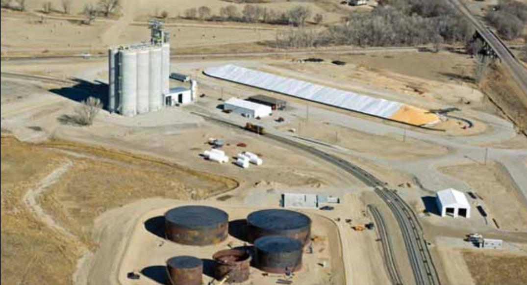
*Aerial view of the Benkelman terminal shows 760,000-bushel slipform concrete elevator and a 2-million-bushel Union Iron Works temporary storage pile, Aerial photo by Heavens View Photography, Sterling, CO.*
