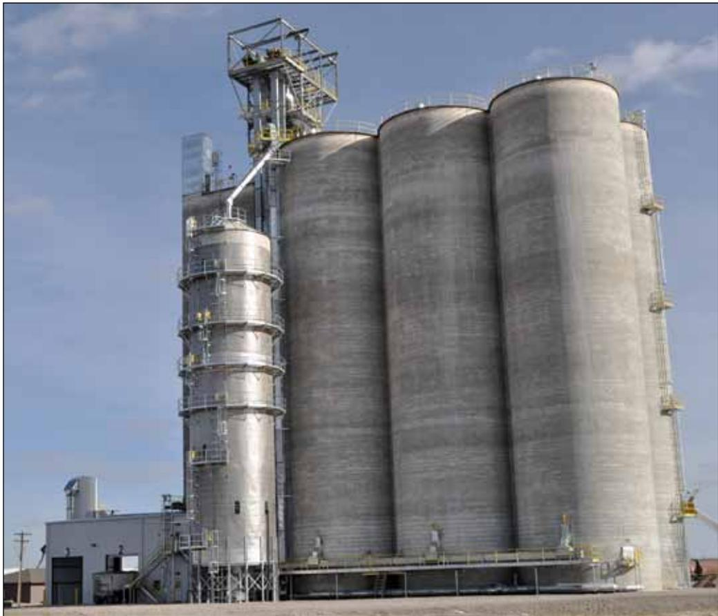
*Ground-level view of the new Gavilon Grain rail terminal elevator in Benkelman, NE, which includes a 760,000-bushel slipform concrete storage structure and a 6,000-bph Zimmerman tower dryer. Ground-level photos by Ed Zdrojewski.*
