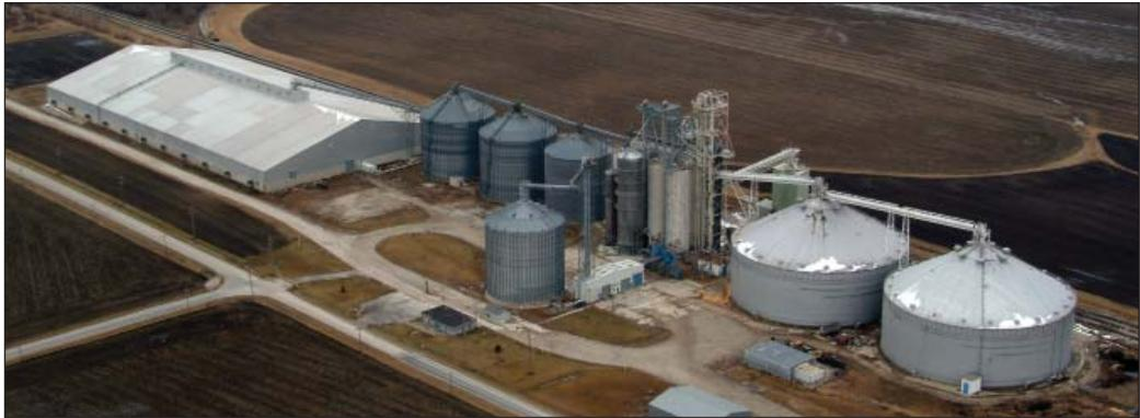
*Prairie Central's rail terminal north of Pontiac, IL. New 10,000-bph Zimmerman dryer is visible near the center of the photo.*
