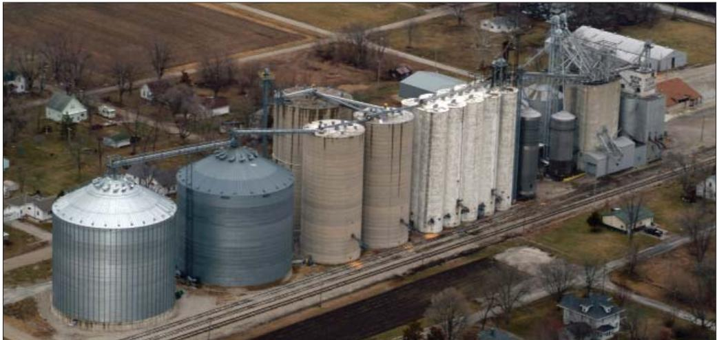
*Prairie Central Cooperative's headquarters elevator at Weston, IL. Top of a new leg is visible behind a large jumpform concrete tank near the center of the facility. Aerial photos by Steve Huey, Pekin, IL.*
