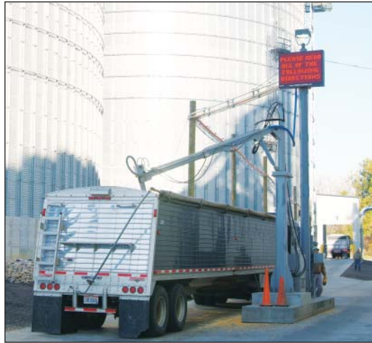
Incoming truck is sampled with a new Intersystems probe prior to dumping at one of two receiving pits in the background. Photo by Ed Zdrojewski.
