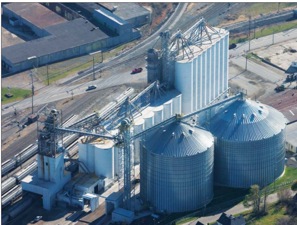
Aerial view of the Town & Country Cooperative rail terminal in Mansfield, OH, with two newest corrugated steel tanks in foreground and a new receiving leg immediately to the left. Aerial photo by Focal Plane Photography, South Euclid, OH
