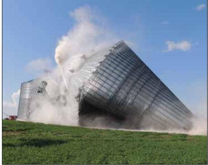
*Damaged 105-foot-diameter tank at left following an Aug. 4 windstorm at the Kentland elevator. At right, the tank is being pulled down by three Caterpillar track hoes pulling steel cable. Storm damage photos courtesy of Grain Flo Inc.*
