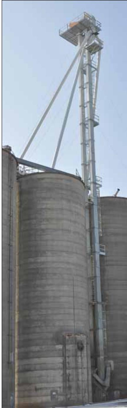
*New GSI 15,000-bph receiving leg is the first of four legs to be replaced at Kentland.*
