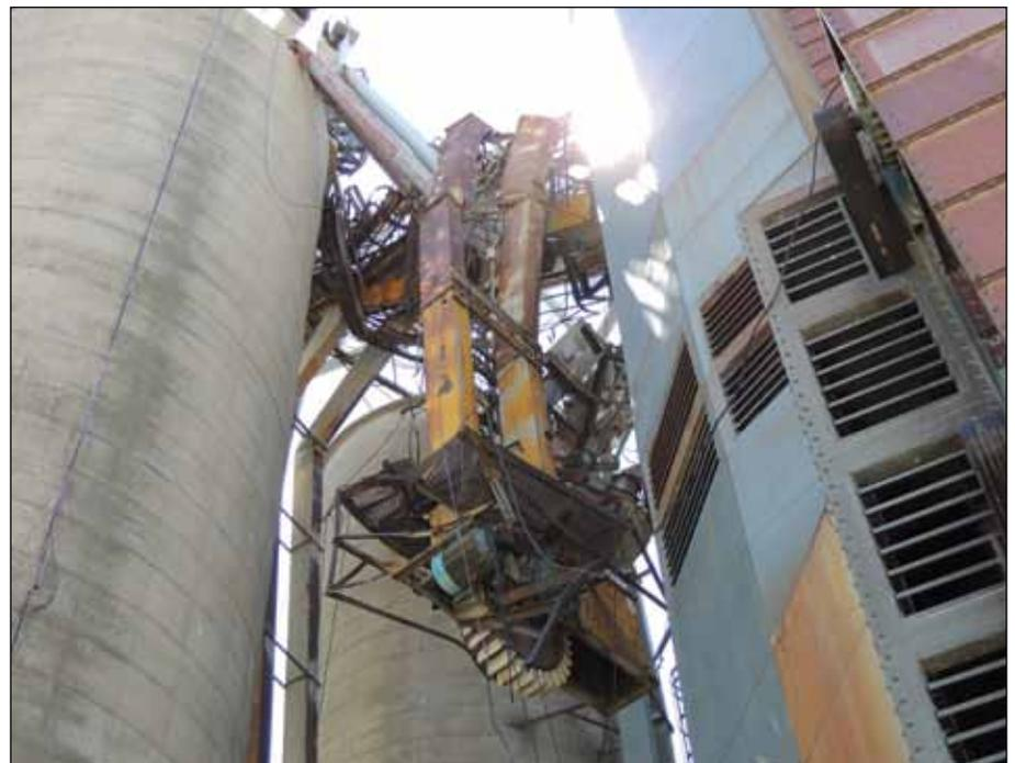
*Damaged 15,000-bph leg hangs down from an overhead catwalk following the Aug. 4 storm.*
