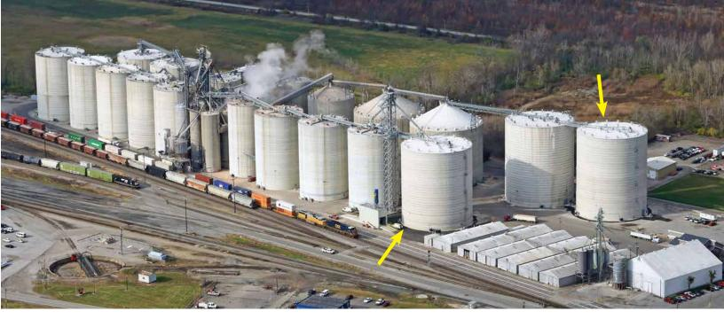
In addition, Central States added a natural gas-fired Zimmerman tower dryer rated at 10,000-bph, the facility's third dryer, bringing total drying capacity to 18,000 bph. The dryer is serviced by 15,000-bph InterSystems wet and dry legs equipped with single rows of 16x8 Tiger-Tuff buckets on 18-inch belts. The dryer had not been used as of *Grain Journal's* visit early in September 2015 but was expected to be fired up for the fall harvest.
