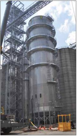
New 10,000-bph Zimmerman tower dryer is nearly completed in September 2015 adjacent to a LeMar tower encasing new InterSystems bucket elevators. Photo by Ed Zdrojewski.
