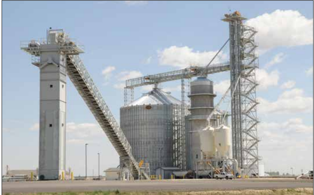
CHS Connell Grain's new 2.2-million-bushel corn elevator in Bruce, WA. It includes a 1.5-million-bushel LeMar temporary storage pile with J & D center fill tower at left. Photos by Bruce Selyem.
