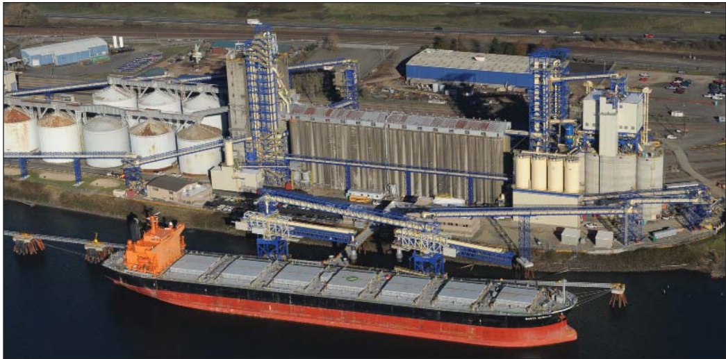
Aerial view of the TEMCO LLC export terminal on the Columbia River at Kalama, WA. New shipping bins are visible at the far right. Aerial photo courtesy of TEMCO.
