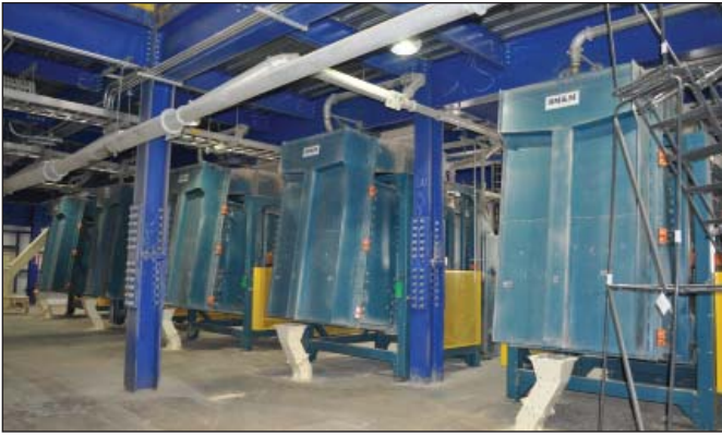
BM&M gyrotory screeners are a part of the cleaning house flow to bring grain up to export standards on FM.
