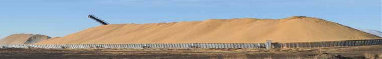
One of two 2-million-bushel temporary storage piles with four-foot LeMar sidewalls, this one holding 2012-crop corn.
