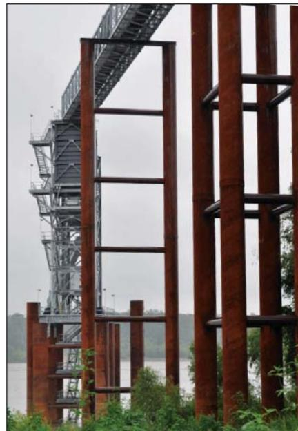
*Half-mile-plus-long covered belt conveyor in a 10-foot Warrior box bridge runs out to the river-side, where a Warrior stair tower over the water supports a Warrior/Micada surge bin and a Premier Fabrication loadout spout (not visible).*
