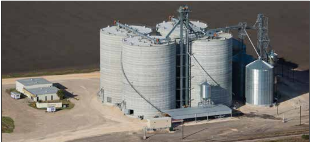
Planter's Grain Cooperative's newly rebuilt 2.7-million-bushel grain elevator adjacent to U.S. Highway 181 between Sinton and Taft, TX. Aerial photo by Red Wing Aerial Photography, courtesy of Hoffmann Inc., which constructed the jumpform concrete silos.
