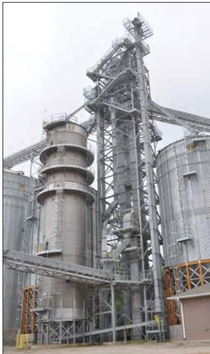
*At left, a 4,000-bph Zimmerman tower dryer. At right, twin GSI 24,000-bph receiving legs, 30,000-bph jump leg, and five-hole Hayes & Stolz swing-type distributor are enclosed by a Warrior support tower with switchback stairs.*
