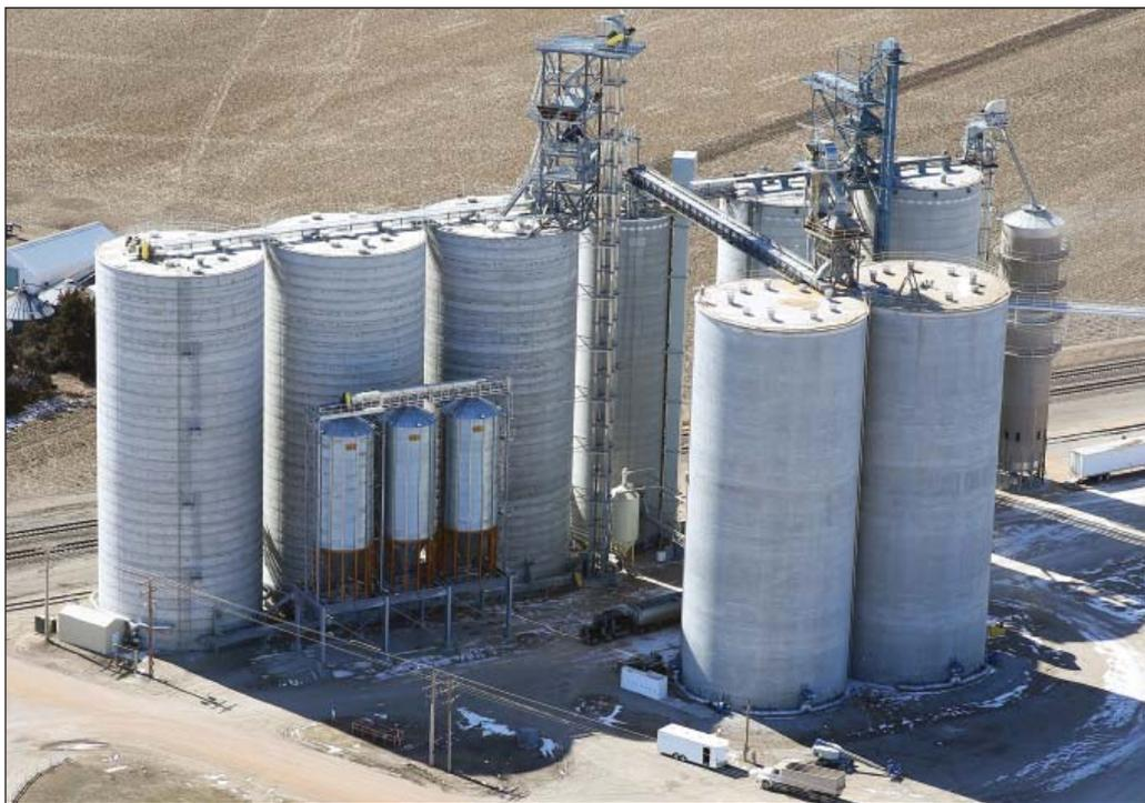
*Aerial view of Aurora Cooperative's grain elevator at Sedan, NE. New construction for 2014 shown in the left half of the elevator includes three new Hoffmann jumpform concrete silos, three new GSI surge tanks, and two InterSystems legs. Aerial photo courtesy of Dakota Aerials.*
