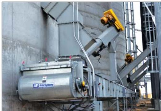
*Telescoping augers coming out of three new 330,000-bushel silos emptying onto an InterSystems 30,000-bph enclosed belt conveyor.*
