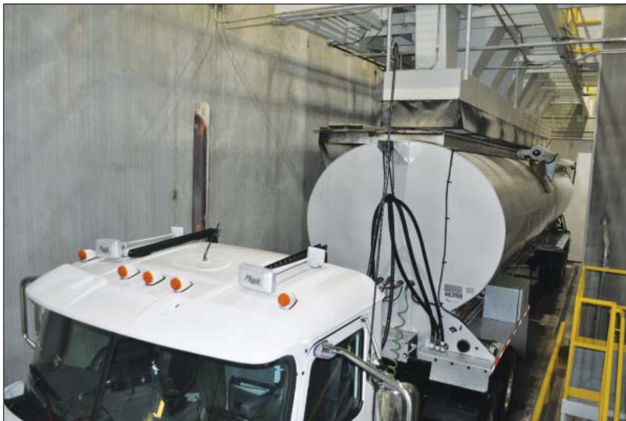
Feed truck is loaded by a Tramco loadout conveyor while parked on a Rick Lake truck scale.
