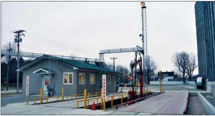
New office building at Clyde and adjacent inbound and outbound truck scales outfitted with a CompuWeigh SmartTruck truck traffic management system.
