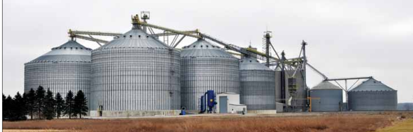
Sunrise Cooperative's 8.4-million-bushel rail terminal at West Clarksfield, OH. A new Behlen 1.1-million-bushel steel tank is the foremost tank in the photo, and a new 1,000-bushel receiving pit with Donaldson-Torit baghouse dust control system is visible in the center of the photo.
