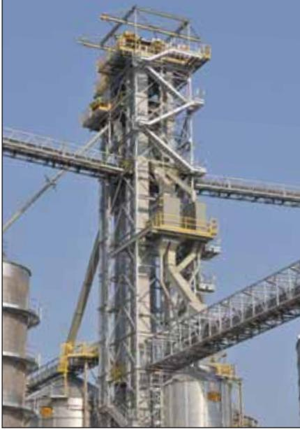
*Closeup of the facility's LeMar center tower including 40,000- and 20,000-bph GSI legs, five-hole Hayes & Stolz rotary double distributor, and a pair of Magik Kleener gravity screeners.*
