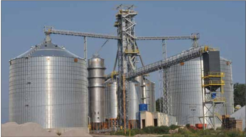
*Auburn Bean & Grain Co.'s new 1.75-million-bushel rail-loading elevator at the edge of Standish, MI including two 730,000-bushel GSI tanks, two GSI grain dryers, and a 40,000-bph CompuWeigh bulkweigher. Photos by Ed Zdrojewski.*
