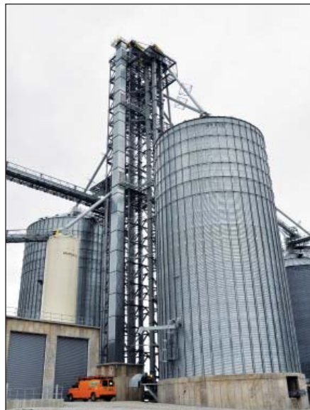
An enclosed manlift provides access to the top of multiple legs serving wet and dry bins.
