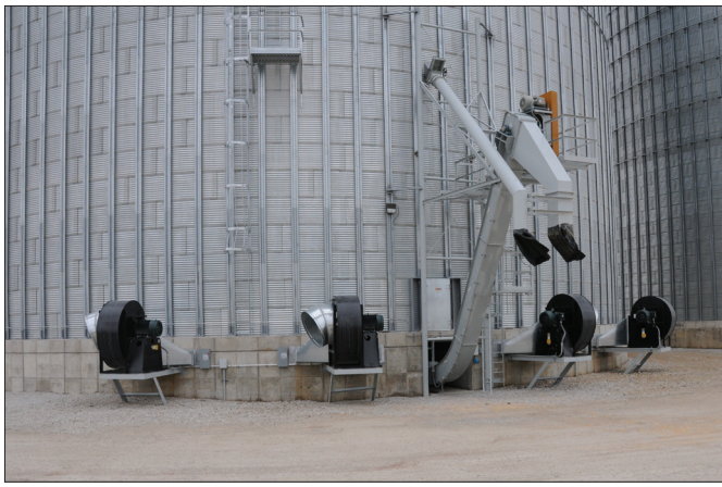
Farmers Cooperative's new GSI 788,000-bushel steel tank is equipped with four Decatur Aeration 60-hp fans and a 15,000-bph GSI reclaim conveyor. Ground-level photos by Tucker Scharfenberg.
