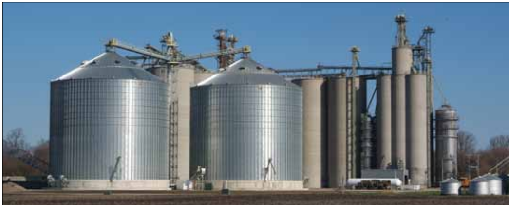
Co-Alliance LLP rail terminal at Scircleville, IN, with two new 691,000-bushel GSI steel tanks at left. Photos by Ed Zdrojewski.
