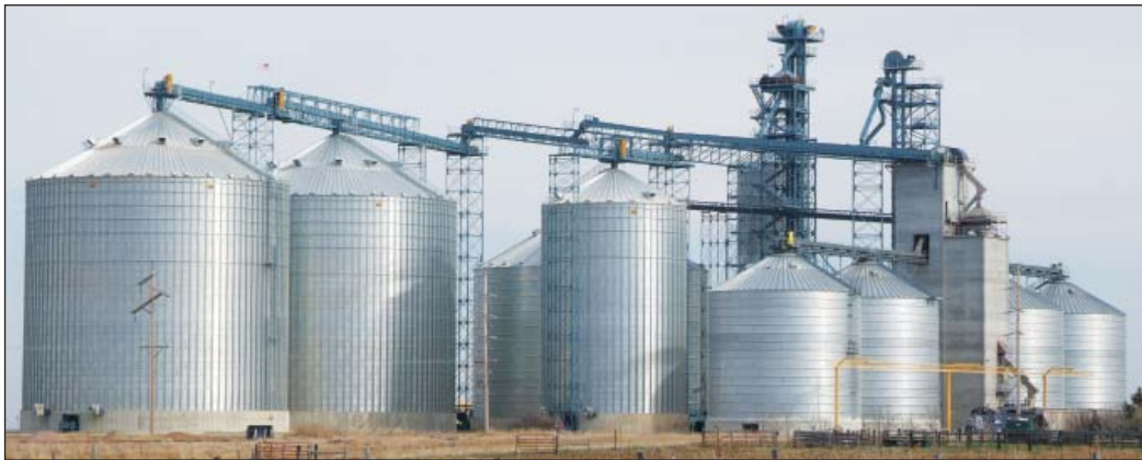
The South Dakota Wheat Growers grain elevator near Highmore, SD, with two new 730,000-bushel storage tanks at left and a new 230,000-bushel wet tank at center. Photos by Ed Zdrojewski.
