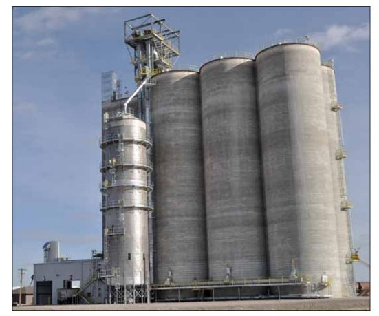
Ground-level view of the new Gavilon Grain rail terminal elevator in Benkelman, NE, which includes a 760,000-bushel slipform concrete storage structure and a 6,000-bph Zimmerman tower dryer. Ground-level photos by Ed Zdrojewski.
