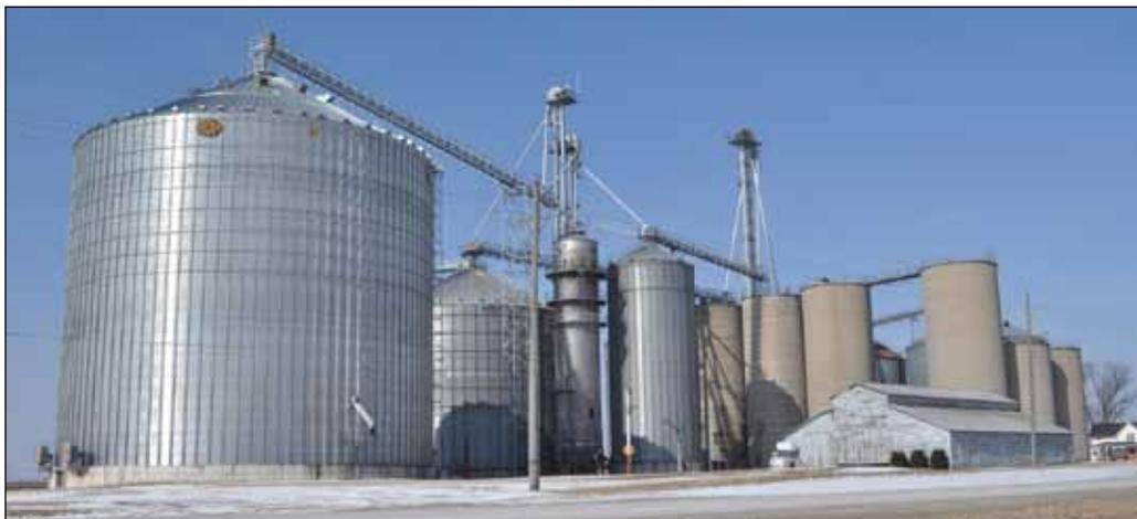
*GRAINCO FS elevator in unincorporated Kentland, IL after a storm damaged it severely in August 2012. Completed construction so far includes a 105-foot-diameter GSI tank at left and the farthest right bucket elevator. Completed construction photos by Ed Zdrojewski.*
