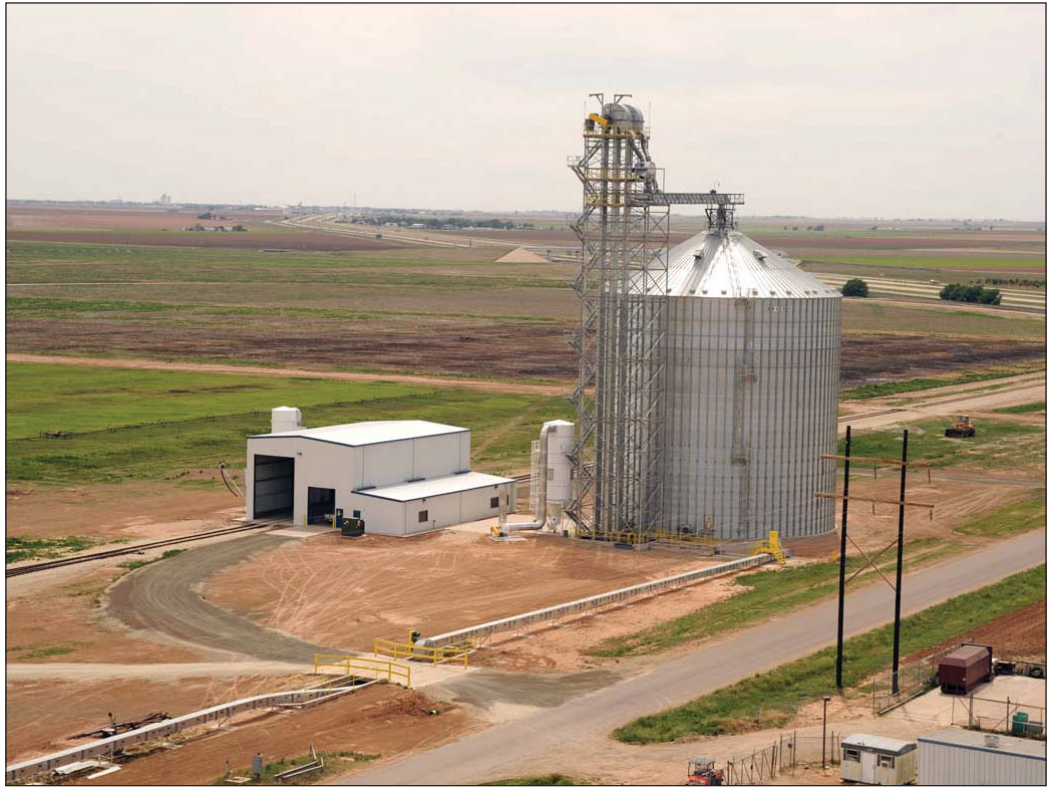
Azteca Milling LP's new 550,000-bushel rail receiving elevator, built in 2008 at its masa plant near Plainview, TX, reputedly the world's largest masa plant, Photos by Bobby's Photography, Plainview.
