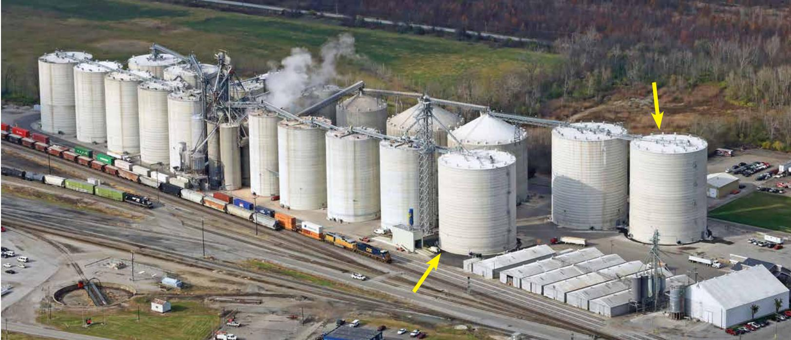
In addition, Central States added a natural gas-fired Zimmerman tower dryer rated at 10,000-bph, the facility's third dryer, bringing total drying capacity to 18,000 bph. The dryer is serviced by 15,000-bph InterSystems wet and dry legs equipped with single rows of 16x8 Tiger-Tuff buckets on 18-inch belts. The dryer
