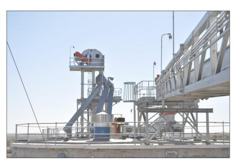
Rooftop equipment, above, includes the head section of a Schlagel 20,000-bph receiving leg and four-hole Schlagel distributor, as well as a 20,000-bph Schlagel drag fill conveyor. At left, a new 1,000-bushel enclosed receiving pit feeds grain into the receiving leg.
