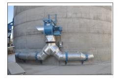
Each tank is equipped with two 40-hp AIRLANCO centrifugal fans plus a 5-hp roof exhauster for aeration at 1/11 cfm per bushel on coarse grains. Two of the tanks have additional 30-hp fans and one a 50-hp fan for air-assisted unloading.
