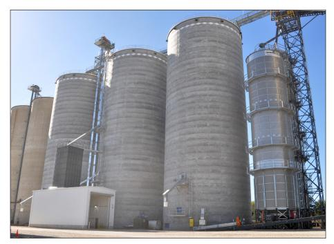
Closeup view of three new McPherson jumpform concrete tanks, receiving pit, and Schlagel leg, and a Brock 4,700-bph tower dryer (not pictured is a Brock 4,000-bph dryer). Ground-level photos by Ed Zdrojewski.
