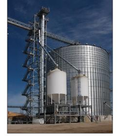
Ground view showing 15,000-bph Schlagel receiving leg in a 16-foot-x-16-foot LeMar tower, six-hole Schlagel rotary distributor, and two 4,000-bushel Meridian surge tanks.
