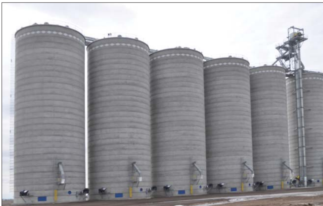
Six new jumpform concrete tanks and a new leg and distributor at far right were added in 2014 at Garden City Cooperative's Lowe elevator northwest of Garden City, KS. Ground level photos by Ed Zdrojewski.
