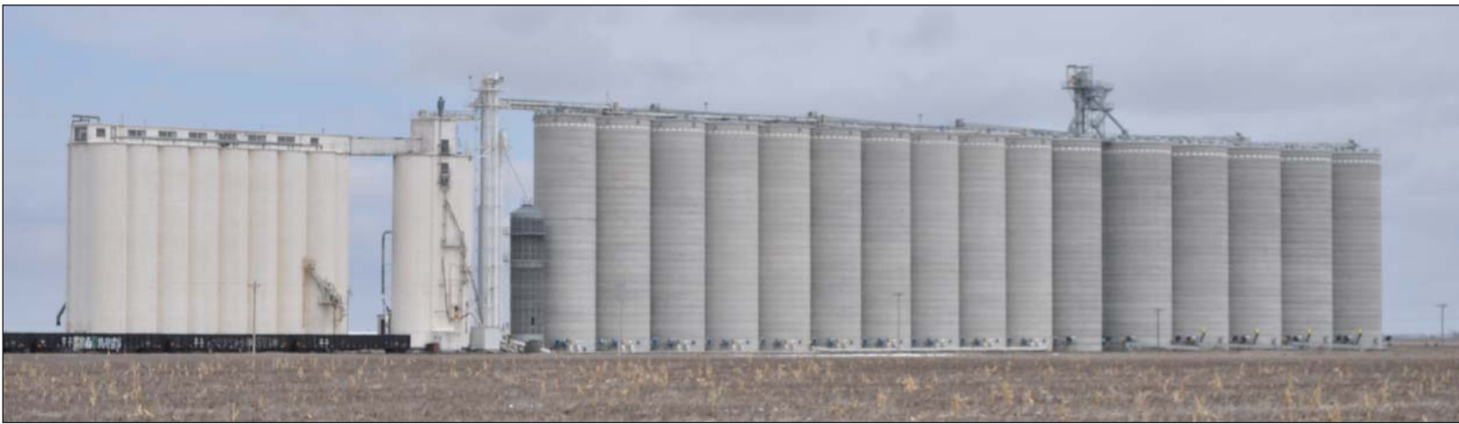
Long-distance view of the Lowe elevator, which holds 2.26 million bushels.
