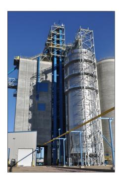
Grain handling equipment, from left, includes a slipform concrete loadout tower; three InterSystems receiving legs, two rated at 20,000 bph and one at 40,000 bph, in a Warrior tower; and 10,000-bph Zimmerman grain dryer.
