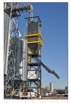
New 50,000-bph CompuWeigh bulk weigh loadout scale is designed for loading both containers and covered hopper railcars. Brock 40,000-bushel hopper tank is visible to the left of the bulkweigher.
