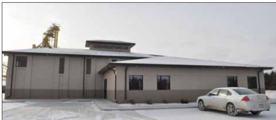
Newly expanded office building includes another 3,500 square feet of space.
