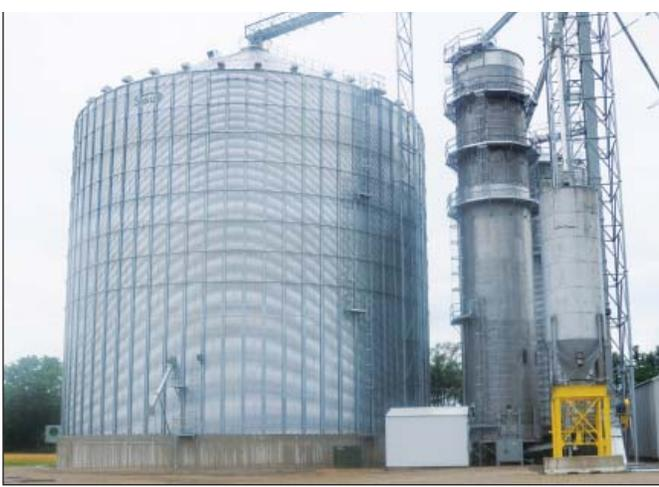
*Sukup 4,700-bph tower dryer to the right of a Sukup 710,000-bushel steel tank. Ground level photos by Tucker Scharfenberg.*
