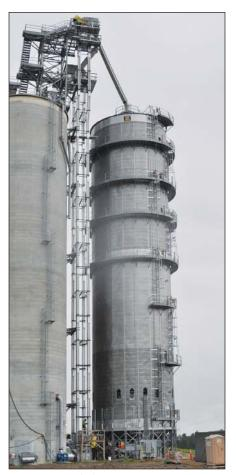
New 12,000-bph Zimmerman continuousflow tower dryer, the largest that manufacturer makes, is serviced by 15,000-bph InterSystems wet and dry legs.
