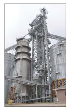
At left, a 4,000-bph Zimmerman tower dryer. At right, twin GSI 24,000-bph receiving legs, 30,000-bph jump leg, and five-hole Hayes & Stolz swing-type distributor are enclosed by a Warrior support tower with switchback stairs.
