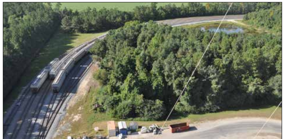
Railyard serving the Bladenboro mill recently was expanded to accommodate 90-car CSX unit trains, up from 65-car trains.
