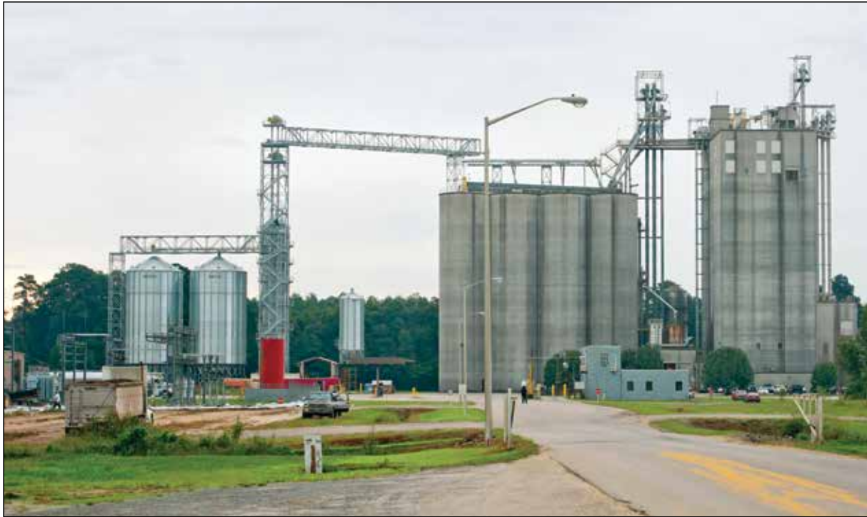
Murphy-Brown's 535,000-tpy swine feed mill outside of Bladenboro, NC, with a new 110,000-bushel wet grain steel annex nearing completion at left. Photo by Lime Light Photography.
