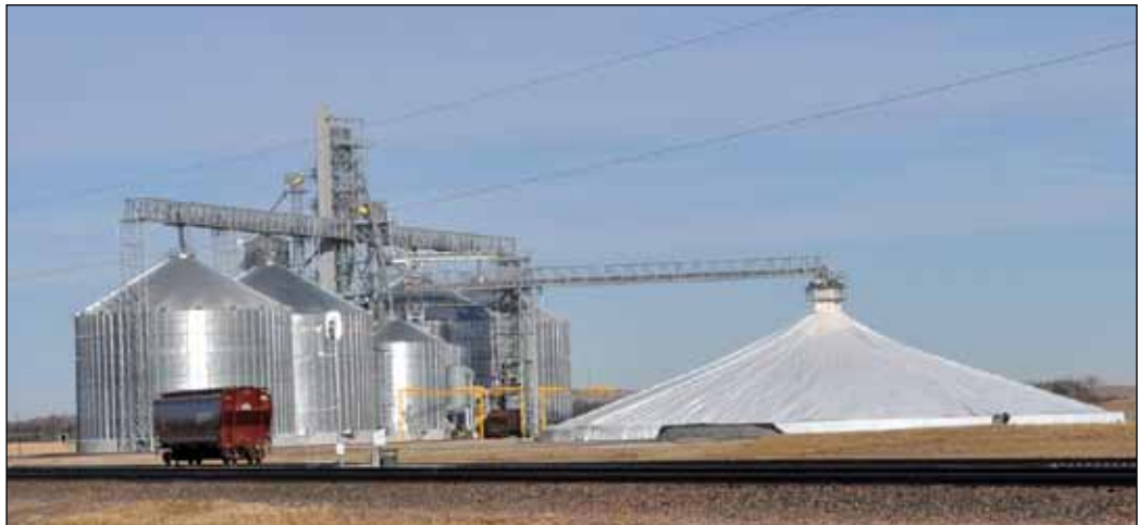
The Andersons' new 4-million-bushel rail terminal outside of Anselmo, NE features 2 million bushels of upright storage, a 2-million-bushel ground pile, and 8,000-foot loop track running off of a Burlington Northern Santa Fe main line. Photos by Ed Zdrojewski.
