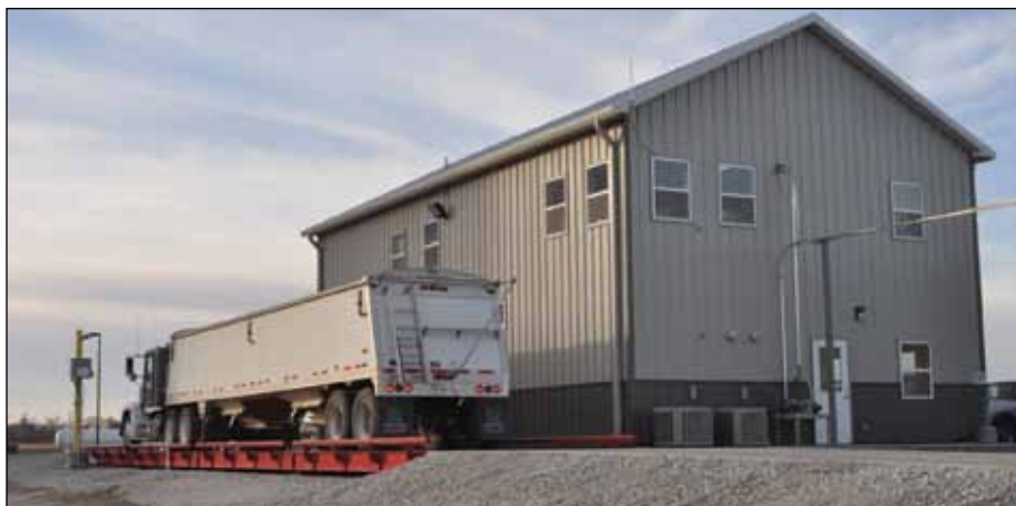
The facility office building sits adjacent to a 90-foot Rice Lake inbound truck scale and Intersystems grain probe. Scales are under control of CompuWeigh software modified by The Andersons.
