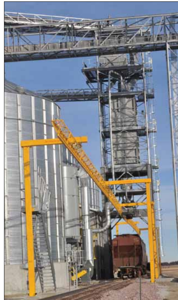
Shuttle trains are loaded by a 60,000-bph Intersystems bulk weigh system topped by a 40,000-bph Intersystems gravity screener all enclosed in an 18-foot-x-18-foot Warrior support tower.
