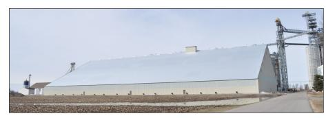
New flat storage building at Ulen, MN was constructed directly over an existing temporary storage pile. It currently can hold 3 million bushels and, with modifications, could hold 3.5 million.
