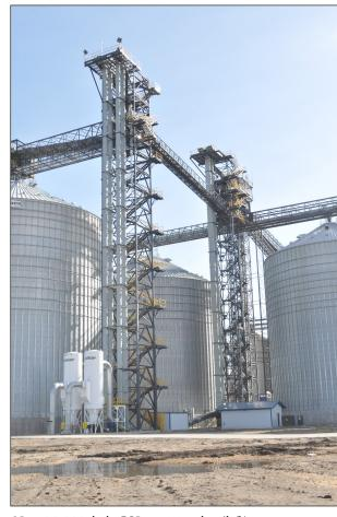
New 20,000-bph GSI receiving leg (left) enclosed in a Warrior tower outfitted with switchback stairs.
