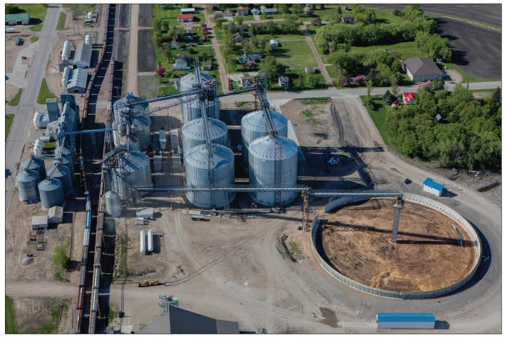
West Central Ag Services added 1.6 million bushels of upright steel storage (tanks at far right) and a 2.6-million-bushel temporary storage pile at its branch elevator in Beltrami, MN.
