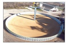
A new 2.6-million-bushel temporary storage system in Beltrami with 16-foot precast concrete walls constructed by Hanson Silo.
