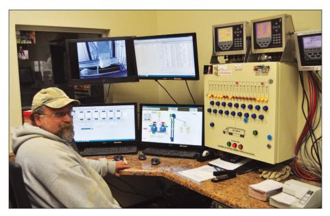
Mill Operator Ken Van Ginkel utilizes an Easy Automation control system to operate the feed mill from a central control room. Ground level photos by Ed Zdrojewski.
