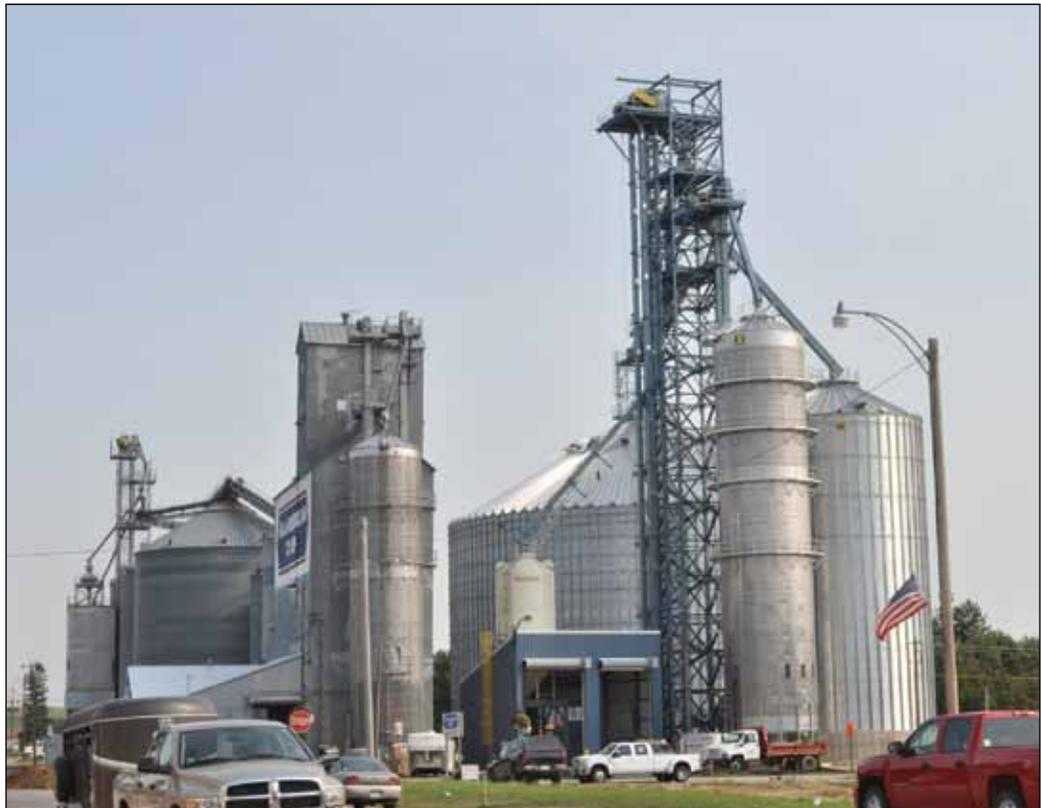
*All American Cooperative's elevator at Elgin, MN with a brand new annex in right half of photo featuring a 1-million-bushel storage tank, 143,000-bushel wet tank, two 20,000-bph receiving legs, and 7,000-bph grain dryer. Photos by Ed Zdrojewski.*
