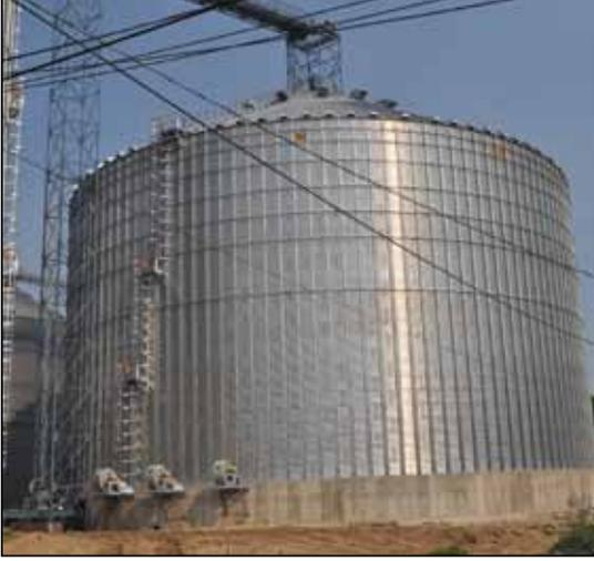
*New million-bushel GSI corrugated steel tank nears completion about a week before the cooperative's open house in September 2012.*
