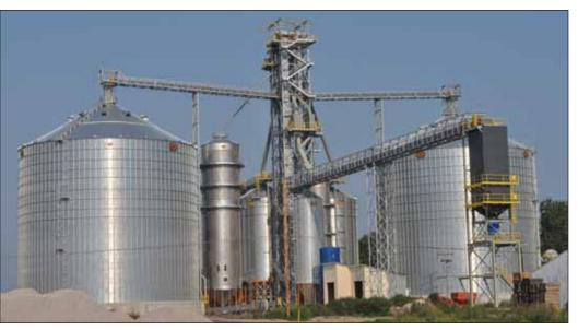
Auburn Bean & Grain Co.'s new 1.75-million-bushel rail-loading elevator at the edge of Standish, MI including two 730,000-bushel GSI tanks, two GSI grain dryers, and a 40,000-bph CompuWeigh bulkweigher. Photos by Ed Zdrojewski.
