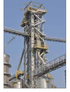
Closeup of the facility's LeMar center tower including 40,000- and 20,000-bph GSI legs, five-hole Hayes & Stolz rotary double distributor, and a pair of Magik Kleener gravity screeners.
