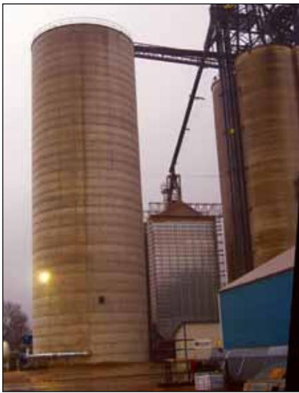
Ground level view of the new wet tank, one of two new dryers, and leg on a rainy November afternoon in central Minnesota. Photo by Ed Zdrojewski.
