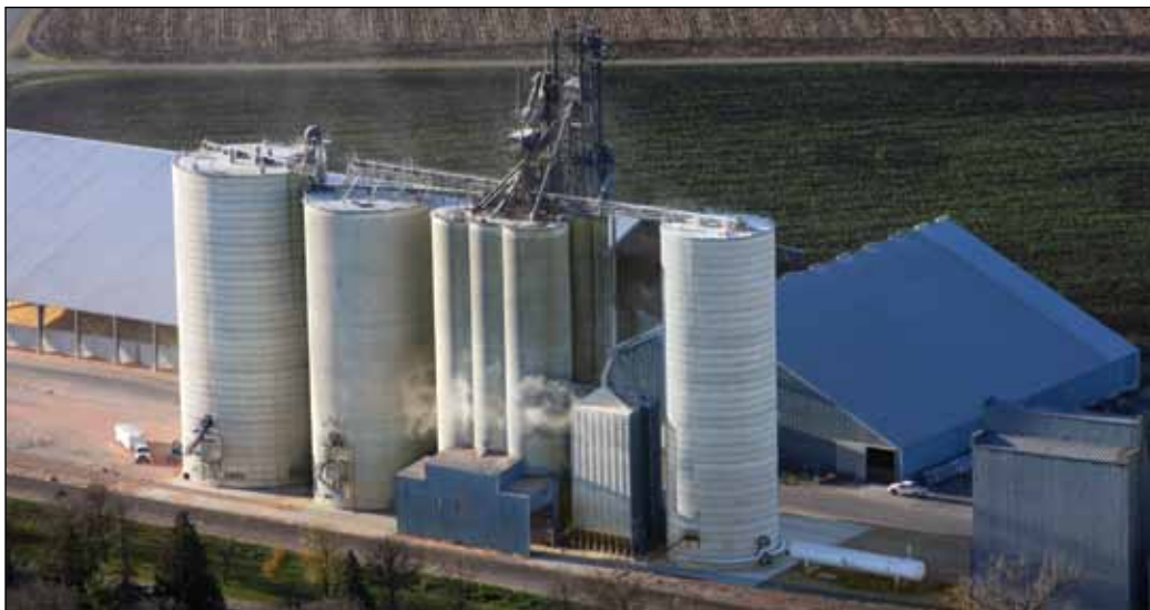
Glacial Plains Cooperative's headquarters elevator in Murdock, MN, has 5 million bushels of upright and temporary storage. A new Hoffmann 220,000-bushel jumpform concrete wet tank and one of two 5,000-bph Grain Handler grain dryer can be seen at right. Aerial photo by JH Photography, Spencer, IA.
