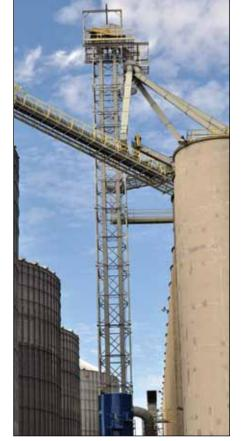
Twin receiving pits and 30,000-bph Hawthorne-Seving receiving leg, which feeds into a six-hole Hayes & Stolz distributor. Photo by Ed Zdrojewski.
