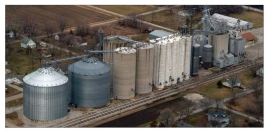
Prairie Central Cooperative's headquarters elevator at Weston, IL. Top of a new leg is visible behind a large jumpform concrete tank near the center of the facility. Aerial photos by Steve Huey, Pekin, IL.
