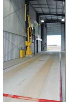
Enclosed scalehouse adjacent to the facility office building includes an 80-foot Rice Lake truck scale, Gamet truck probe, and CompuWeigh SmartView screens.
