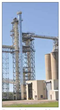
Two new enclosed receiving pits feed a pair of 25,000-bph Essmueller receiving legs enclosed in a LeMar tower.
