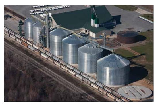
Sunrise Cooperative Inc.'s 3.7-million-bushel rail terminal near Crestline, OH, with a new 1-million-bushel Behlen tank at far right and the concrete foundation for one of two more million-bushel tanks under construction to the right of that. Aerial photo by Focal Plane Photography, South Euclid, OH.
