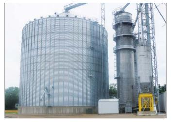
Sukup 4,700-bph tower dryer to the right of a Sukup 710,000-bushel steel tank. Ground level photos by Tucker Scharfenberg.
