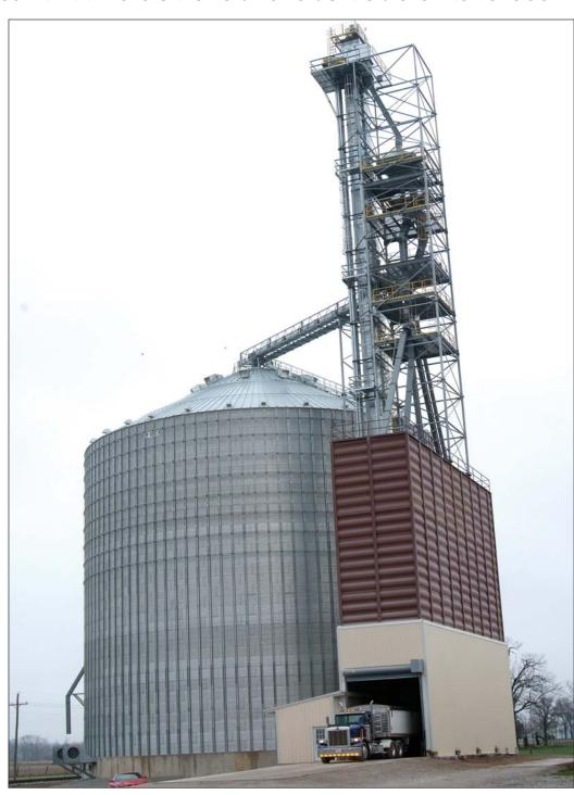
New 735,000-bushel steel annex at the Harvest Land Cooperative elevator in Hagerstown, IN, including, from left, Brock grain storage tank, receiving and loadout shed with four 8,000-bushel plus one 1,500-bushel Baker Rullman square steel bins, and LeMar tower housing a 20,000-bph InterSystems leg, InterSystems gravity cleaner, and two Schlagel distributors. Photo by Ed Zdrojewski.
