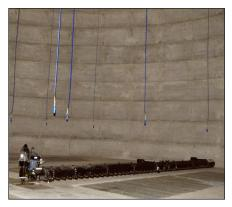
Daay paddle sweep and TSGC grain temperature monitoring cables inside one of the two larger upright storage tanks.
