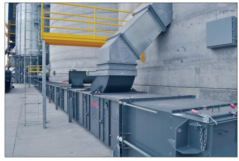
Hi Roller Hi Life reclaim enclosed belt conveyor runs at 60,000 bph.
