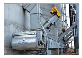
Telescoping augers coming out of three new 330,000-bushel silos empty onto an Inter-Systems 30,000-bph enclosed belt conveyor.
